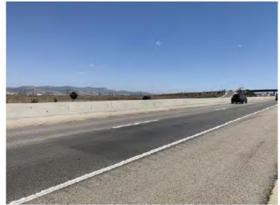
④ Southbound U.S. 101 facing southeast across the project site
