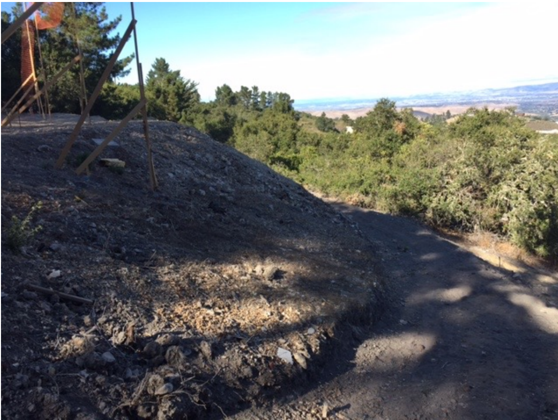
Figure 7. Another view of upper portion of disturbed slope below proposed home building site and narrow road/path that also needs to be restored and/or outsloped. Upon completion of slope shaping and track rolling operations apply native seed mix and erosion control blankets.
