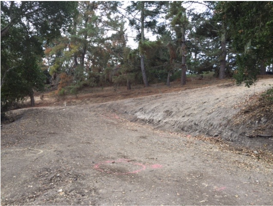
Figure 11. Install rice straw or wood chip mulch in foreground (i.e., flatter areas) and erosion control blankets (e.g., jute net) and straw wattles on steeper slopes (e.g., right of center) to stabilize exposed soil surfaces and prevent erosion problems.
