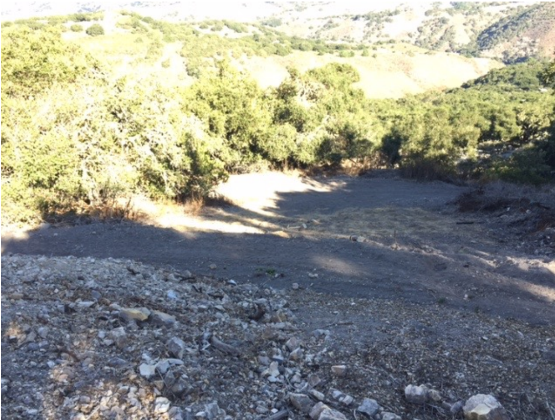
Figure 5. Steep and disturbed slope viewed from building pad seen in last photo is greater than 25% grade. A narrow road/path is located in mid slope and at bottom of slope. Properly shape and track roll slope prior to applying hydromulch and erosion control blankets. Also, install straw wattles (i.e., slope interruption measures) in upper and lower section of slope to assist in stabilizing and protecting impacted slope. The oak tree that was removed was located in foreground in lower center portion of photo.
