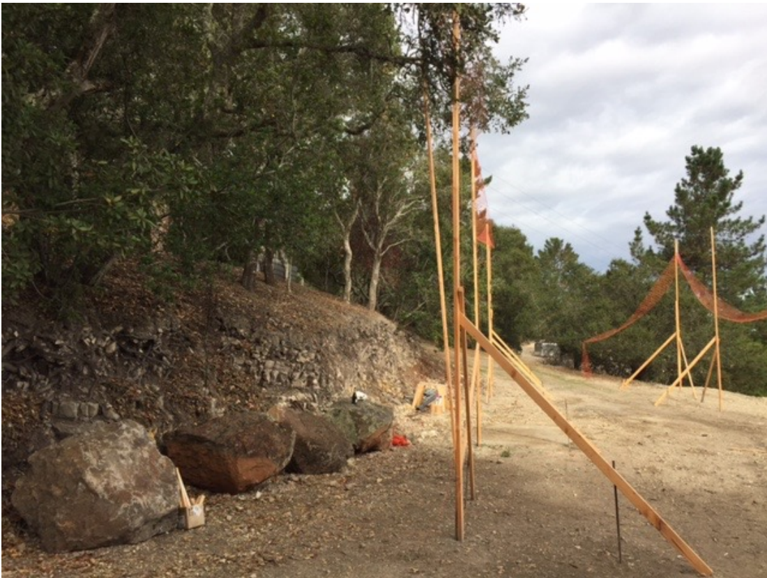
Figure 13. Proposed building pad and site was developed by previous property owner. Relatively immature oak trees located above cut slope are in generally good health and condition and have adapted to the grade change that occurred several years ago. Retain cut slope and building pad/terrace. Install root preservation measures on cut slope (refer to arborist report).
