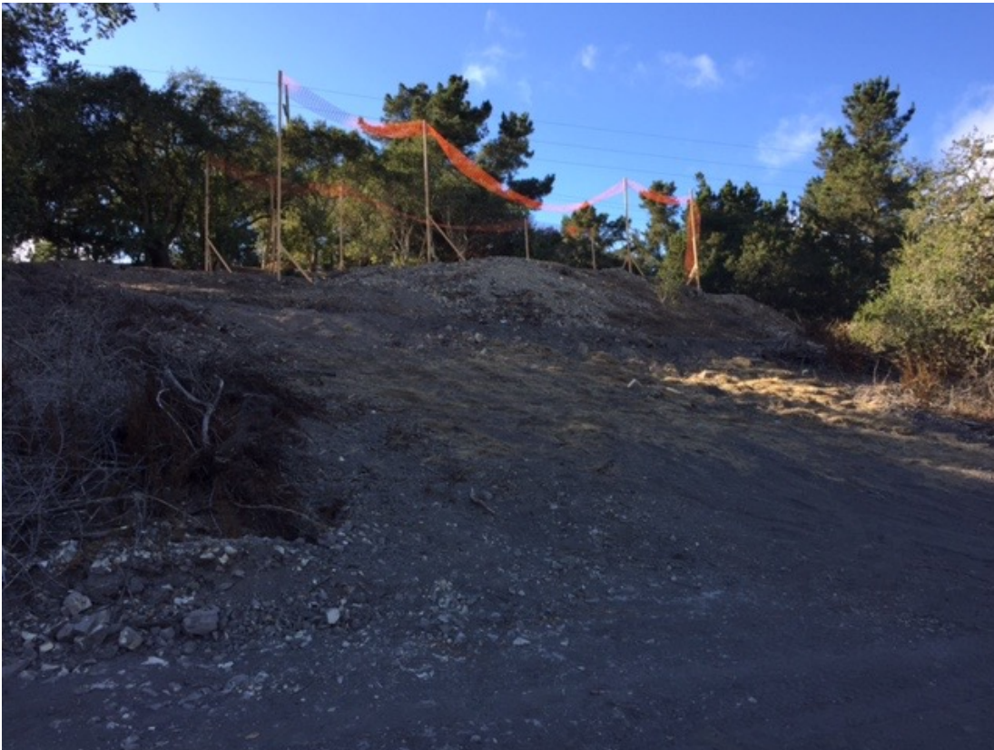
Figure 6. Another view of disturbed and exposed slope below proposed homesite that needs to be stabilized and restored. Oak that was removed was located near top of slope (center portion of photo).
