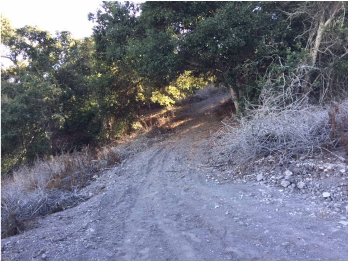
Figure 9. Vertically track roll exposed soil surfaces followed by the application of native seed mix (preferably via hydromulch) and erosion control blankets (e.g., jute net should be sufficient).
