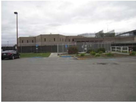
① Existing parking lot where housing addition is proposed (facing north)
