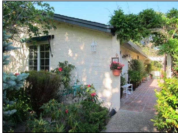
Figure 15. Bldg. 25 constructed of adobe.
