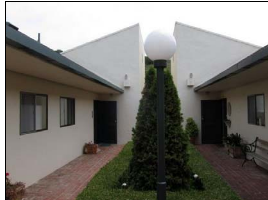
Figure 33. Courtyard of Bldg. 7.
