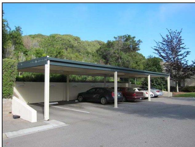
Figure 12. Typical covered parking area.
