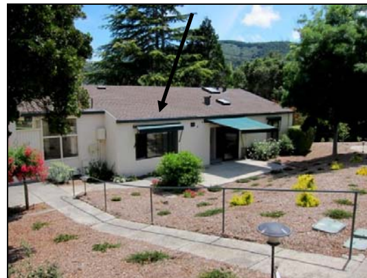
Figure 38. Rear of Bldg. 29 showing garage conversion.
