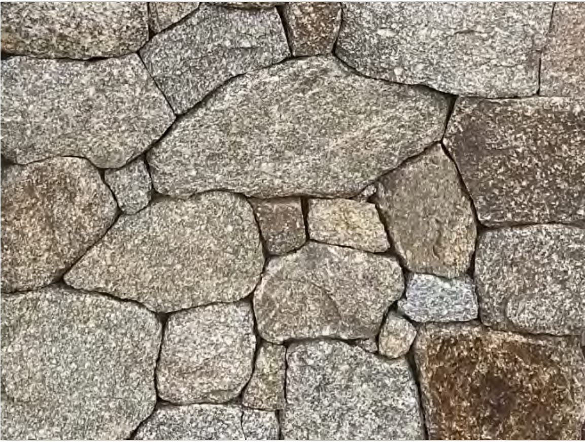
LOCALLY SOURCED, UNCOURSED RANDOM ASHLAR STONE WALLS
