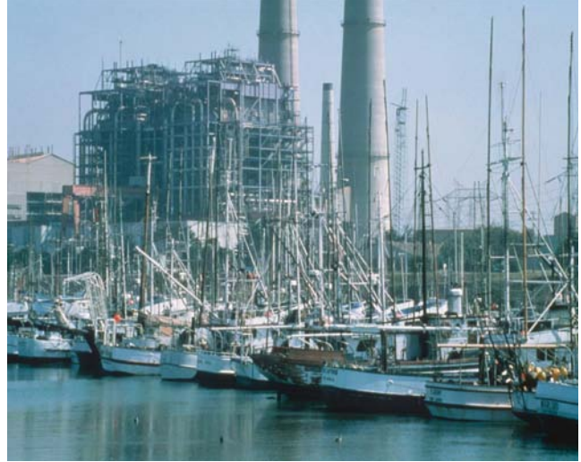
Figure HDD-1 – Moss Landing Harbor
