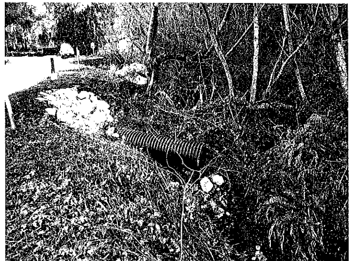
After – Extension of storm drain pipe to carry water to original flow line and riprap fill
