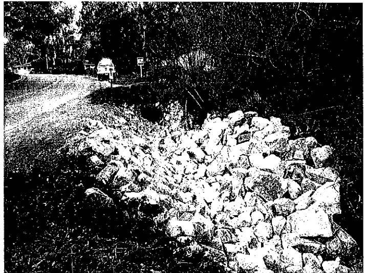
After (looking uphill) – Extension of storm drain pipe and riprap fill
