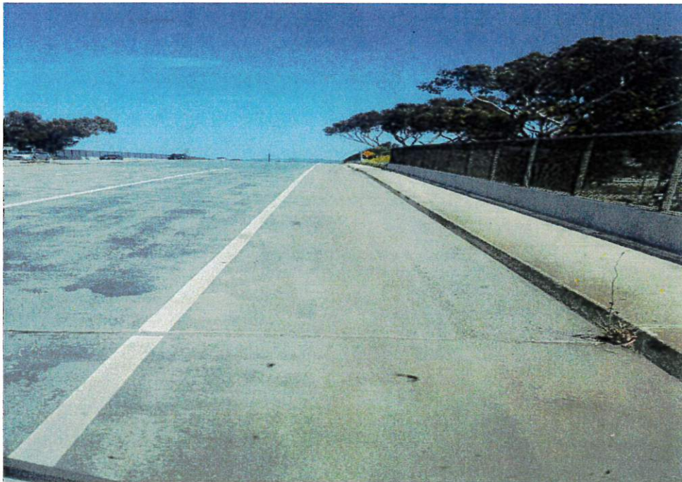
AFTER: Davis Rd. Bridge 5-1-2020 (SAMPLE)
