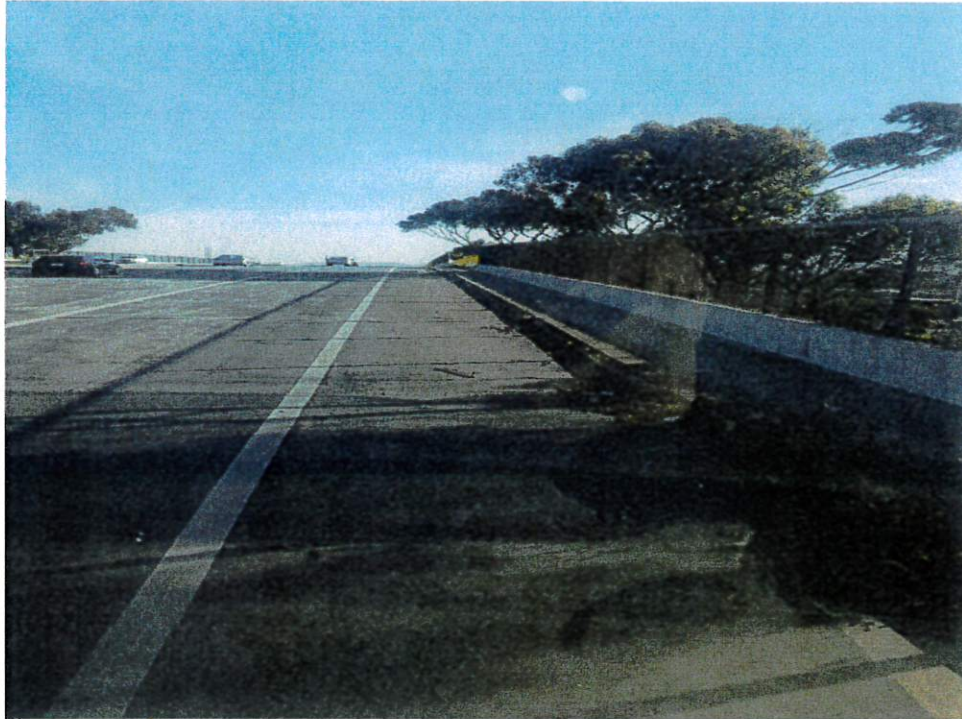
BEFORE: Davis Rd. Bridge 5-1-2020 (SAMPLE)
