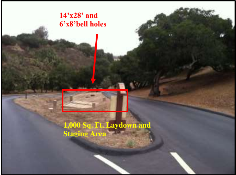
Figure 15. The 14'x28' and 6'x8' bell holes.
