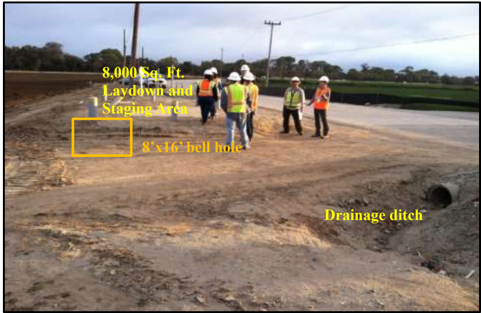
Figure 4. The 8'x16' bell hole and 8,000 Sq. Ft. Laydown and Staging Area.
