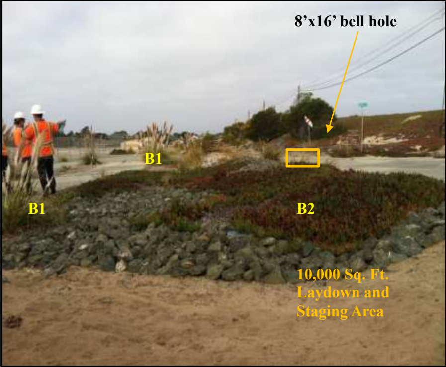
Figure 7. The 8'x16' bell hole and 10,000 Sq. Ft. Laydown and Staging Area.
