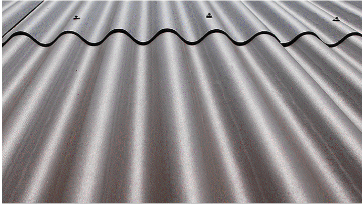
3 NEW GARAGE - EXTERIOR ROOFING
