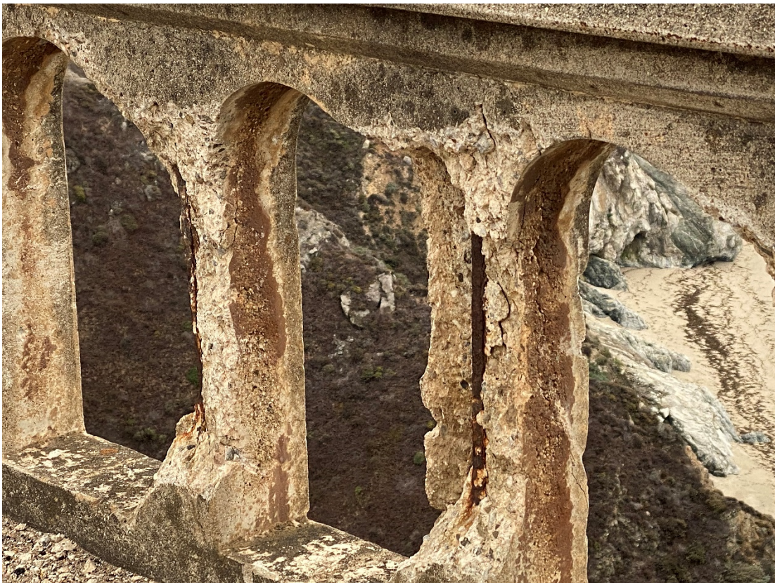
Figure 1-2 Photo of Bixby Creek Bridge Rail Deterioration
