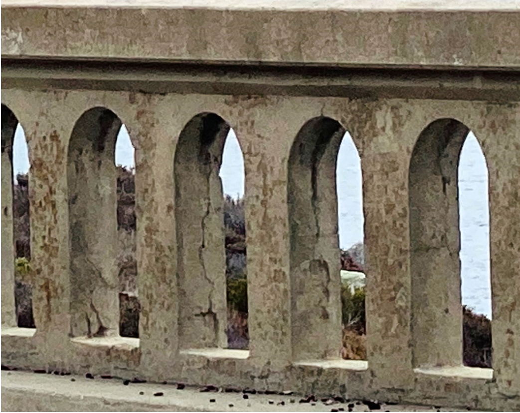
Figure 1-7 Photo of Malpas Creek Bridge Rail Deterioration
