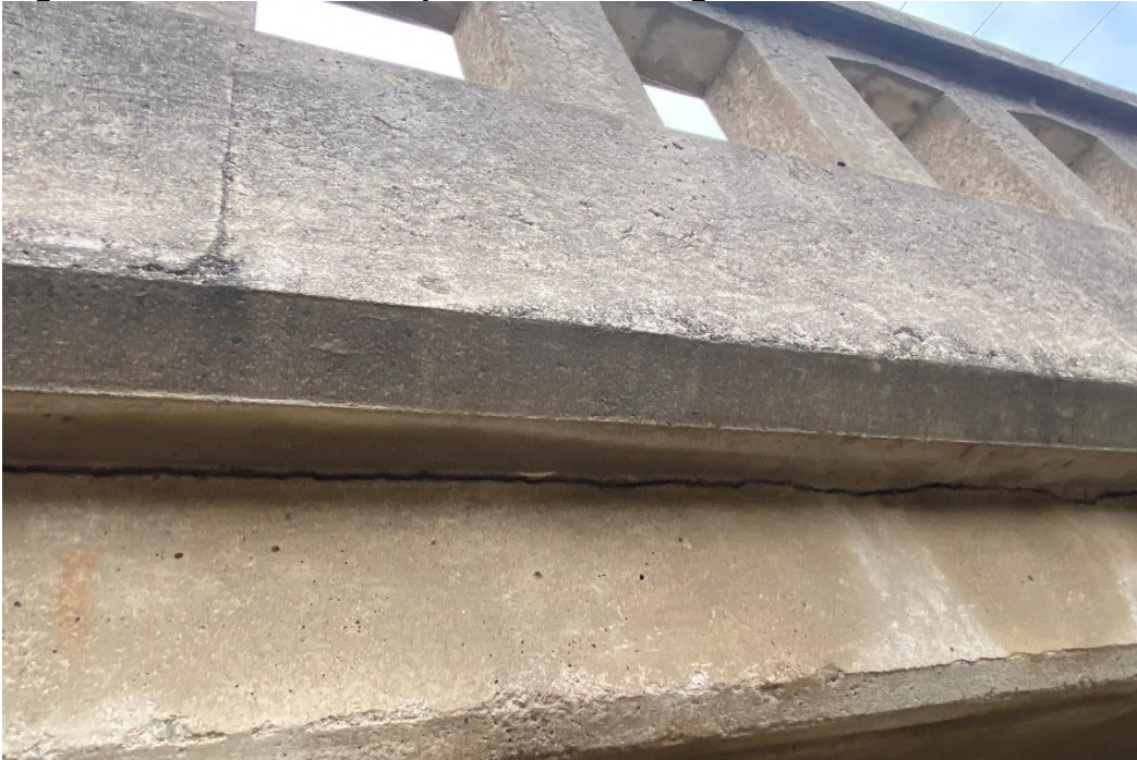
Figure 1-7 Photo of Malpas Creek Bridge Rail Deterioration
