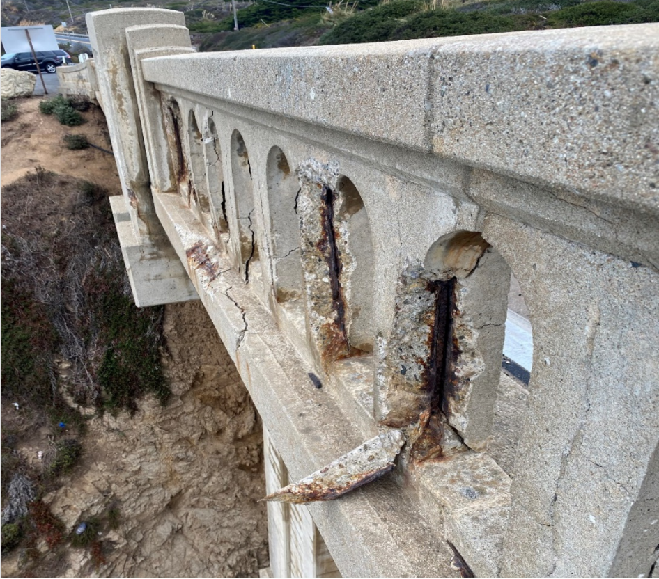
Figure 1-4 Photo of Garrapata Creek Bridge Rail Damage
