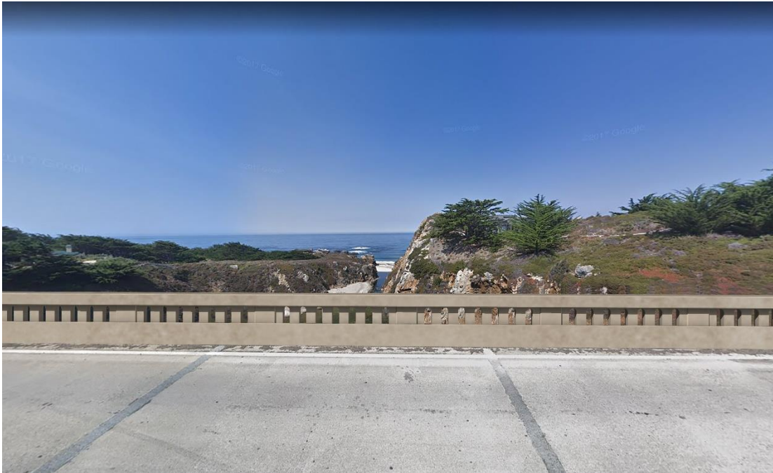
Figure 1-15 Photo Simulation of Barrier Type 86 (front view)
