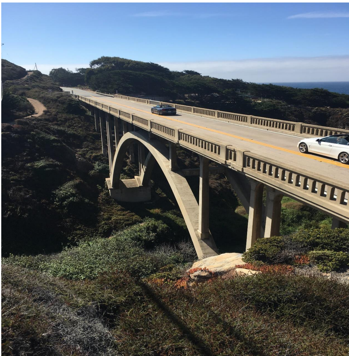
Figure 1-10 Photo of Garrapata Creek Bridge
