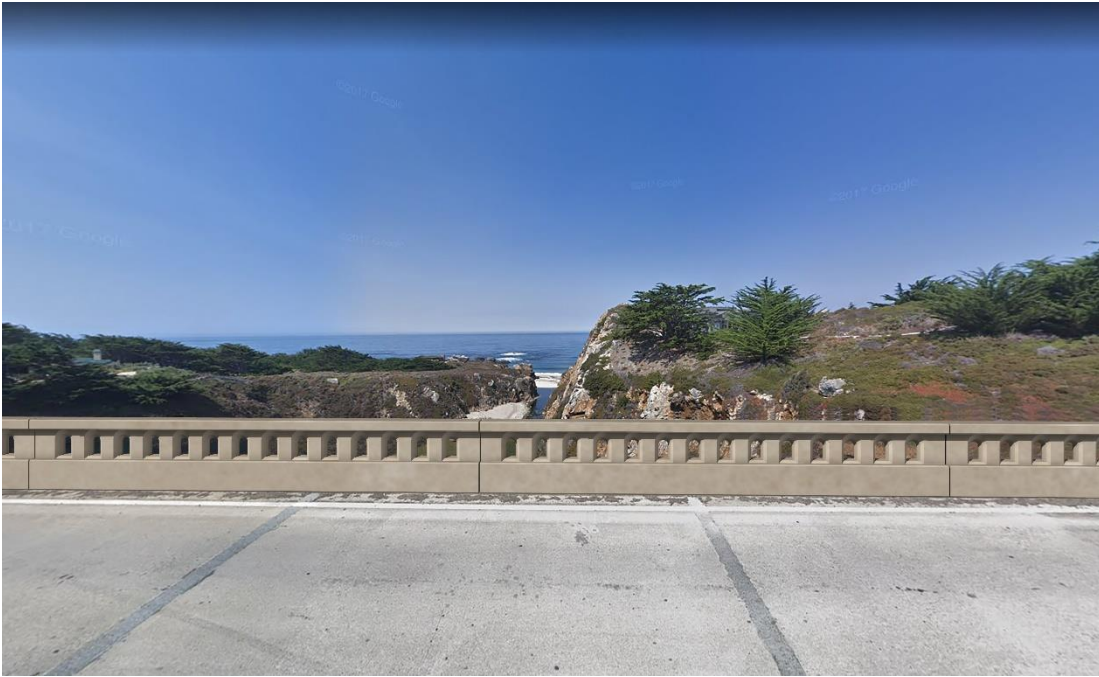
Figure 1-14 Photo Simulation of Barrier Type 86
