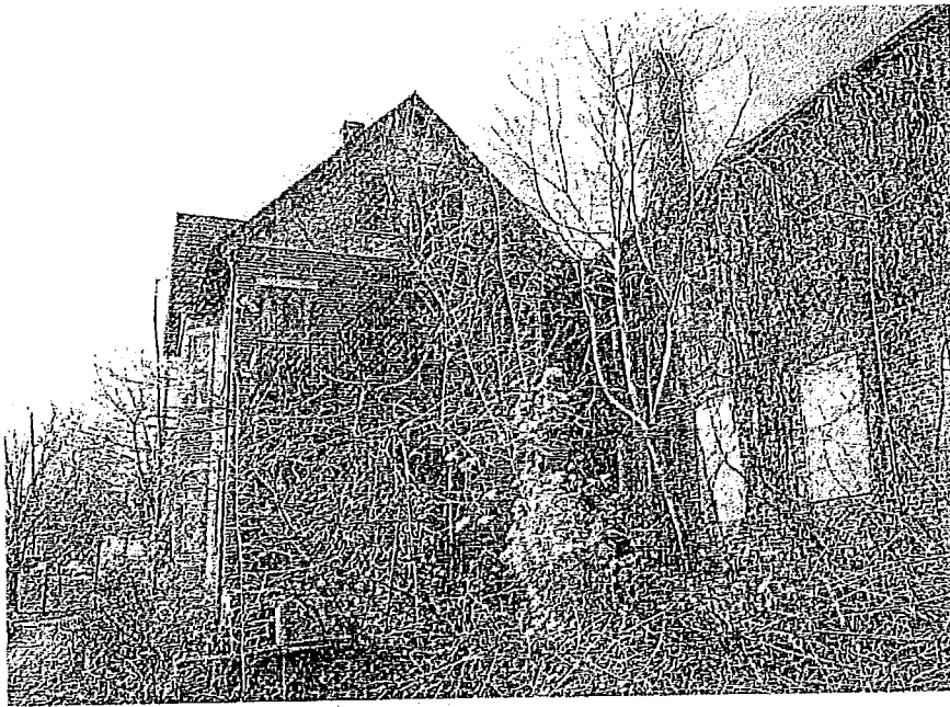
Figure 2. Improper treatment: Boarding up without adequate ventilation, lack of maintenance, and neglect of this property have accelerated deterioration. Photo; NPS file.
