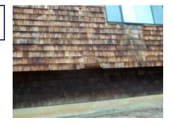
Replace failing cedar siding on lodges at Lake Nacimiento with pest resistant concrete siding. Remove bat infestation and remediate all damage.
