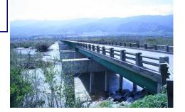
The existing Gonzales River Road Bridge will be replaced with a new bridge approximately 44-feet wide and 1,661-feet long and will be raised to provide for adequate clearance during storm events.
