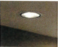
4" LED RECESSED LIGHT FIXTURE BELOW EAVES AND BALCONIES, SALT RESISTANT, APPROX. 9.5 WATTS EA.
