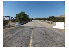
This project includes application of methacrylate to 12 bridge decks and polyester overlay to 4 bridge decks. These bridges are located throughout Monterey County.
