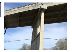
Project entails the placement of scour countermeasures to protect exposed bridge piers 18 and 19. The scour countermeasures will consist of placing rock slope protection (RSP also known as riprap), sheet pile, or other scour-control measures to reduce scour and undermining of structure footings. The footprint of the RSP, sheet pile, or other scour-control measures will extend no further than 100 feet from each bridge face.
