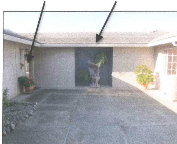
Figures 1 and 2. Left image shows the front elevation, taken from the driveway. The house is built around a front courtyard (arrow). Right image details the front courtyard. An addition with vertical wood siding and shed roof was placed in front of the original wall, the front entrance relocated to the left and the post-adobe construction system removed (arrows).
