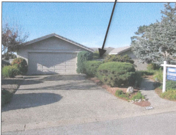
Figures 1 and 2. Left image shows the front elevation, taken from the driveway. The house is built around a front courtyard (arrow). Right image details the front courtyard. An addition with vertical wood siding and shed roof was placed in front of the original wall, the front entrance relocated to the left and the post-adobe construction system removed (arrows).
