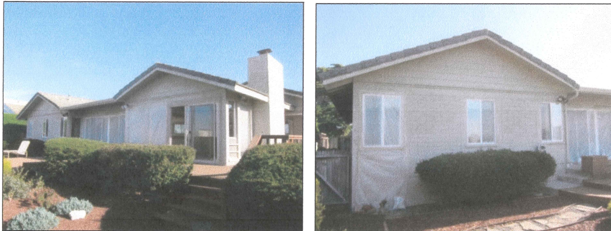
Figures 3 and 4. Left image shows the rear elevation, with painted post-adobe wall material and the additional sliding glass doors. Right image details the rear elevation, with painted post-adobe and replaced windows.
