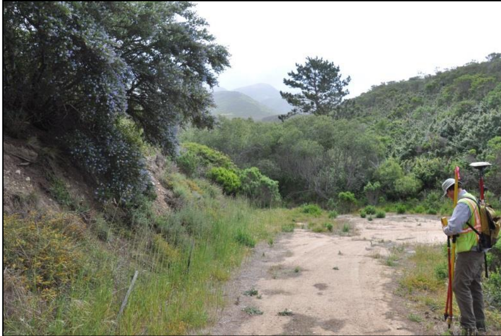
Figure 5 – Access driveway and culvert area over seasonal drainage. May 10, 2012.
