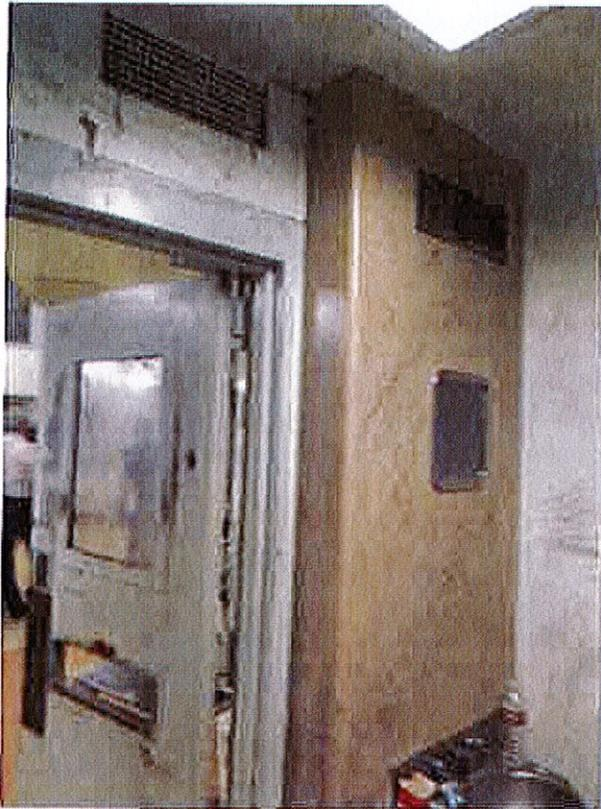
**Men's Housing A and B Pod – Mechanical grills in cells have excessive openings. Return air grill is on the right in photograph.**
