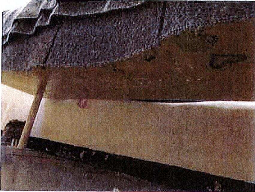
Women's Housing V Pod - View of underside of cell bed in Holding cell showing gap between bed and wall, and inmate graffiti.
