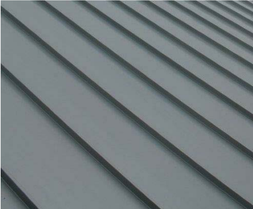
PRE-WEATHERED ZINC STANDING SEAM ROOF
