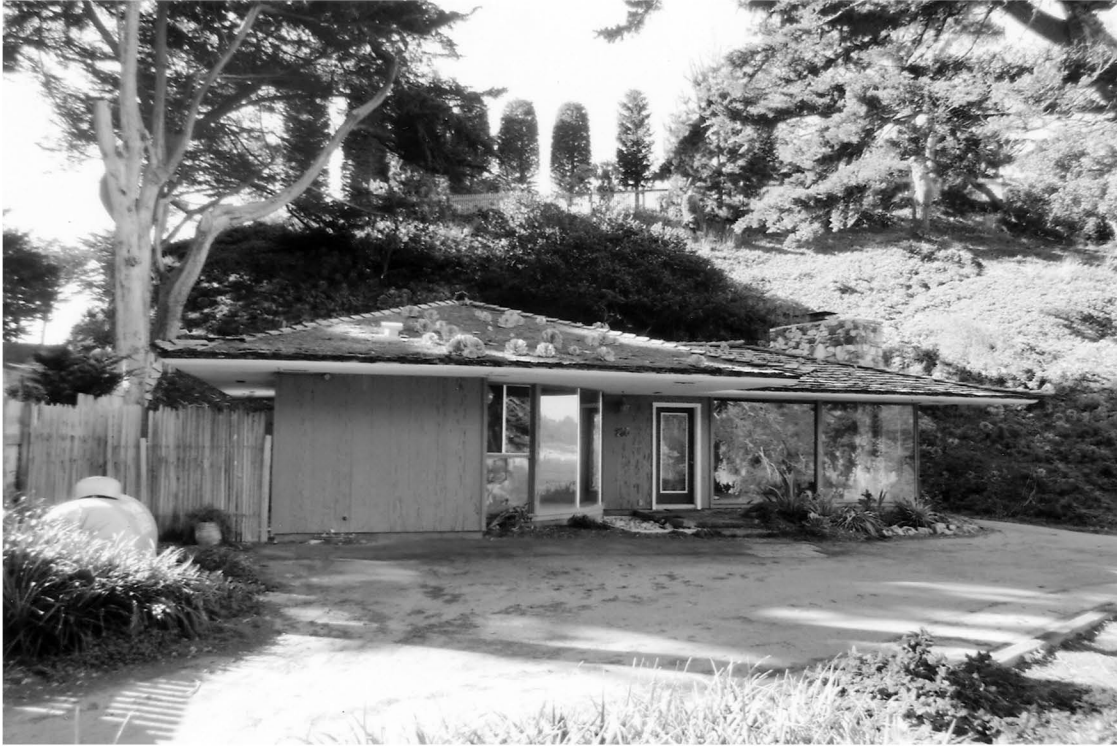
Photo #1. Looking NW at the east facing façade, note the close Proximity of road bed, Kent Seavey, December, 2016.
