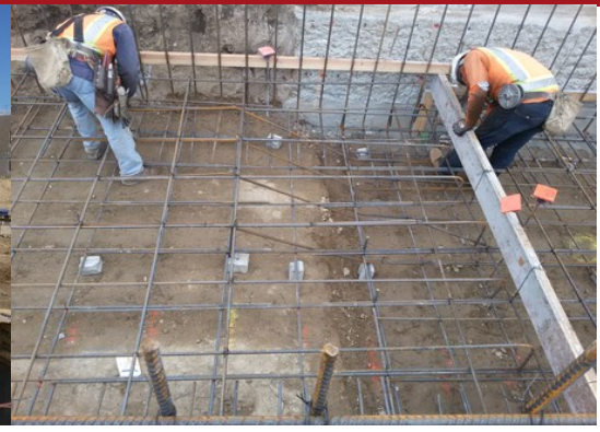
Placing Rebar at Corridor
