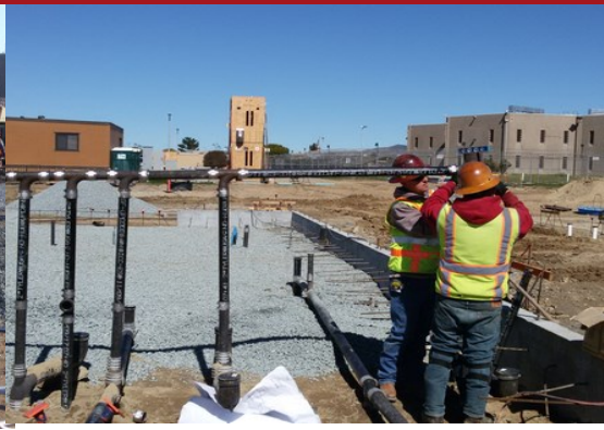
Area C Under Slab Plumbing
