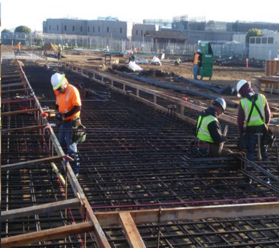
Detention Slab Rebar Placement
