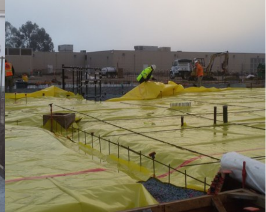
Under slab Vapor Barrier
