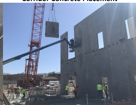
Precast Wall Panel Placement
