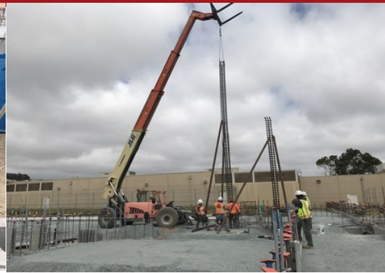
Cast In Place Concrete Columns
