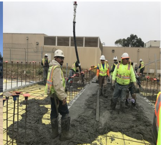
Corridor Concrete Placement
