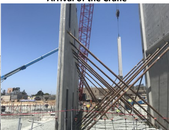
Wall Panel Bracing
