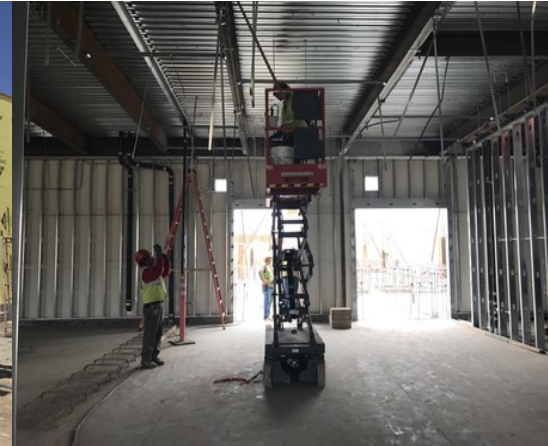
Building A Installing Hangers for MEP
