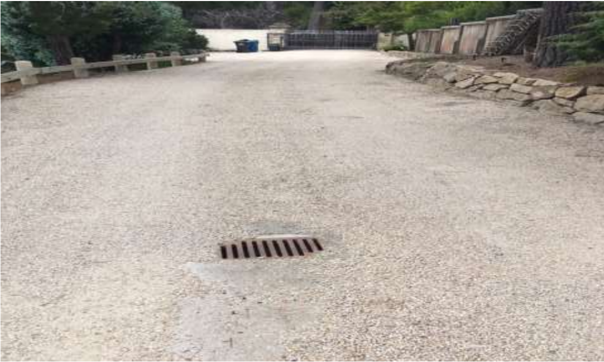
DG and Gravel To Match Existing (gravel and chip seal to be removed and new gravel applied (to match existing)
