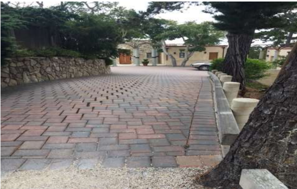
Pavers to be removed, to remove existing chip seal, and pavers re-applied over sand base (to match existing).
