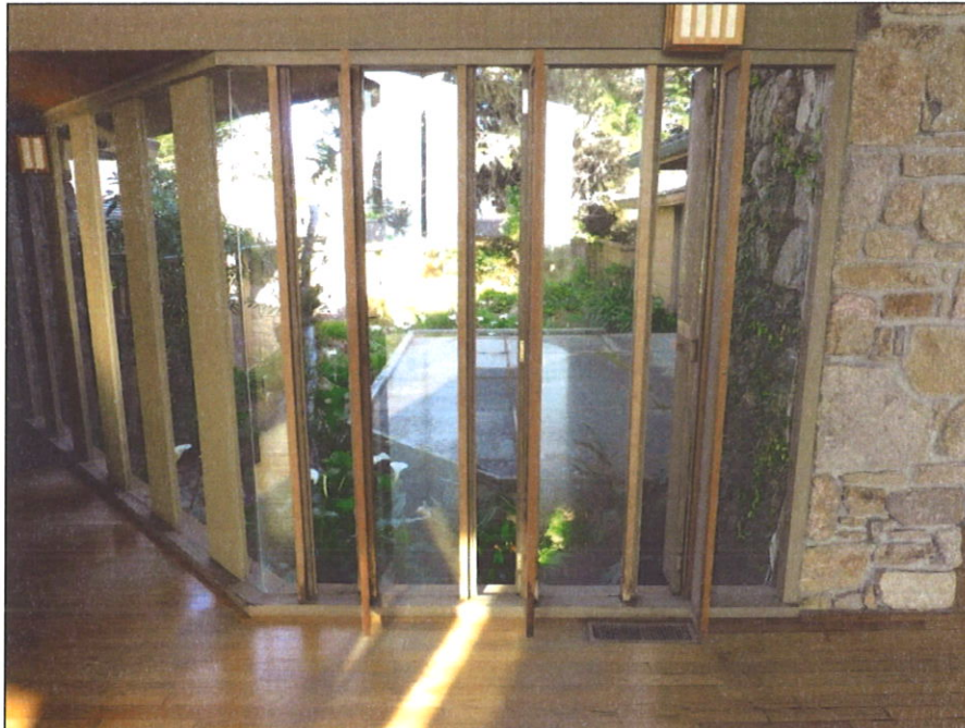
Photograph 26: Detail of three openings permitting passive ventilation. Camera facing east, March 16, 2016.
