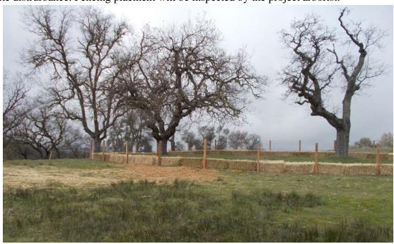
Fencing along the proposed driveway will consist of orange plastic fencing supported by metal "T" posts spaced no further than six feet apart. Straw bales will be placed either behind or in front of the fencing depending on available space. (typical example of fencing and barricades on following page).
