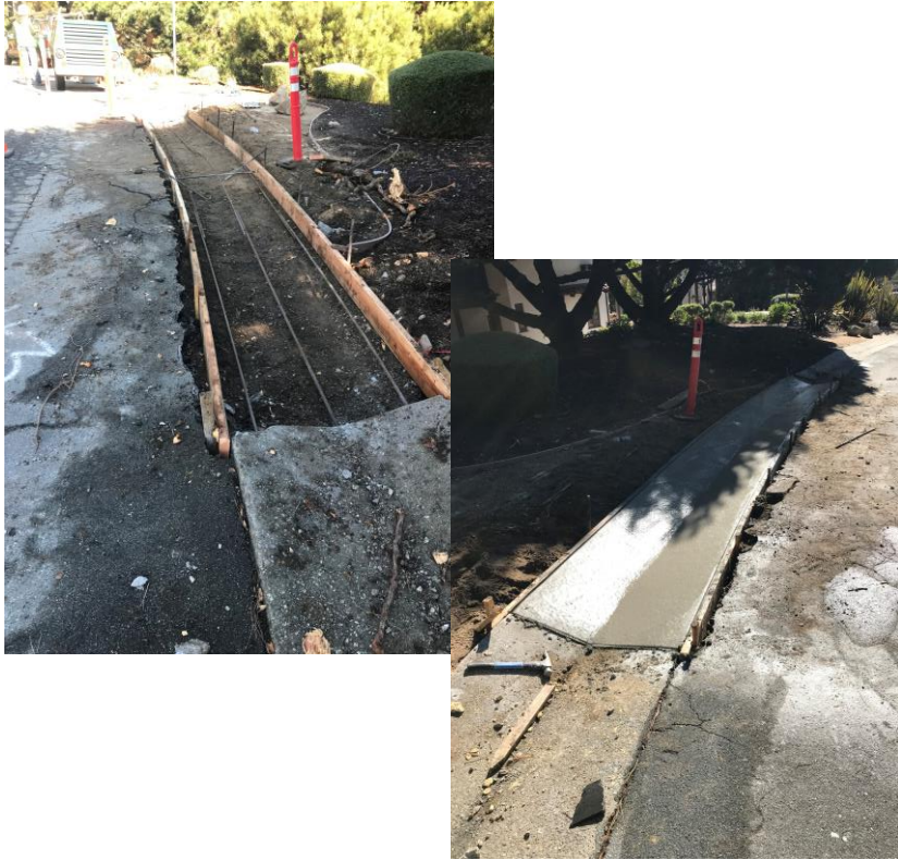
CSA 51 High Meadows Street & Valley Gutter Repair (8 locations)
