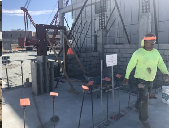
CMU Installation APSI SixthDimension CONSTRUCTION MANAGEMENT
