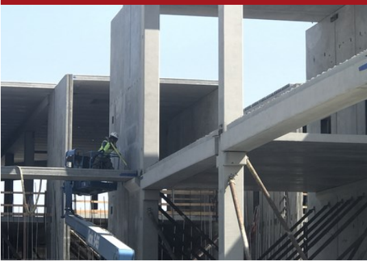
Precast Beam Placement Area C
