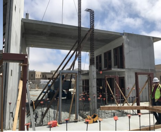
Pre-cast cells with 2nd Tier Deck
