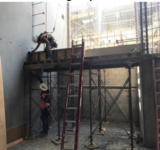
Cast-in-Place Concrete Forms
