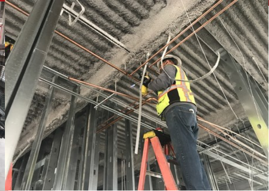
Overhead Plumbing Installation
