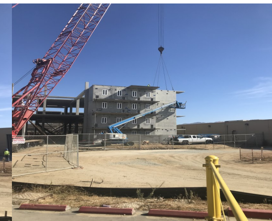
Last Pre-Cast Cell Placed APSI SixthDimension CONSTRUCTION MANAGEMENT
