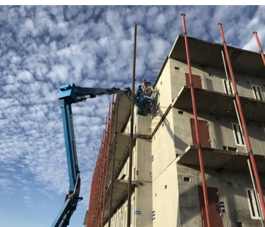
Welding TS to Decks
