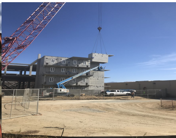
Placing Last Detention Cell
