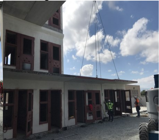
Setting Pre-Cast Cells Area C
