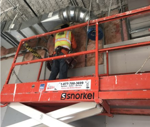
Admin Duct Installation
