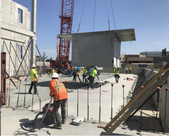
Setting of 1st Pre-cast Cells
