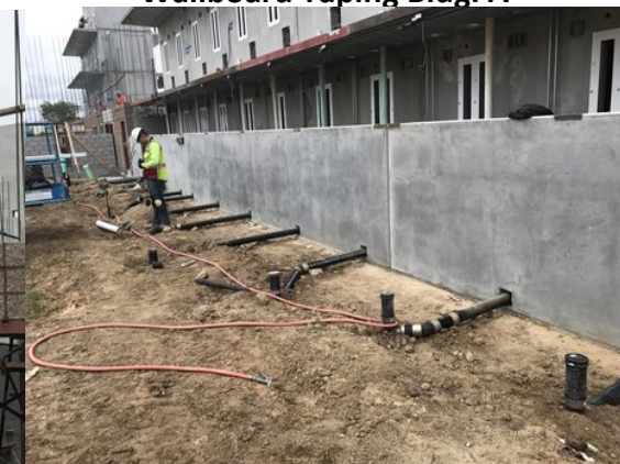
Waste Lines from Detention Cells
