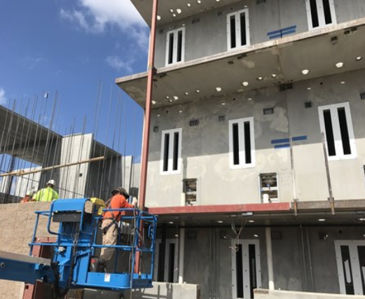
Tube Steel Wall at Chases
