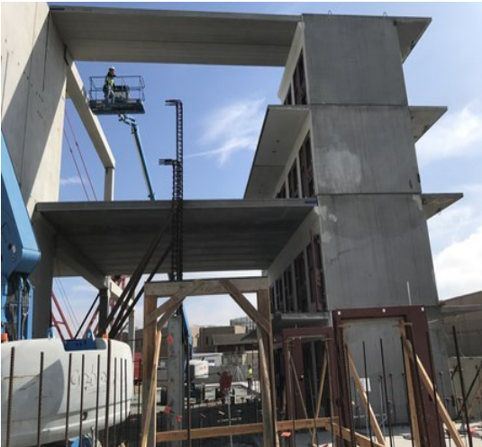
1st and 2nd Tier Pre-cast Cells
