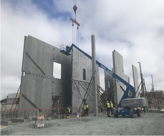
Pre-cast Wall Erection
