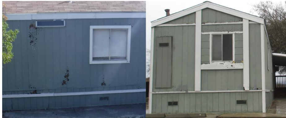
Exterior damage on “employee housing” modular units above Lynch Campground.
