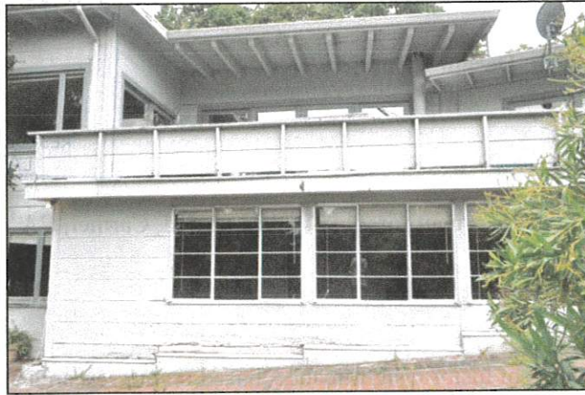
Figure 3. Detail of rear elevation, showing front deck and living space beneath, finished with steel casement windows.
