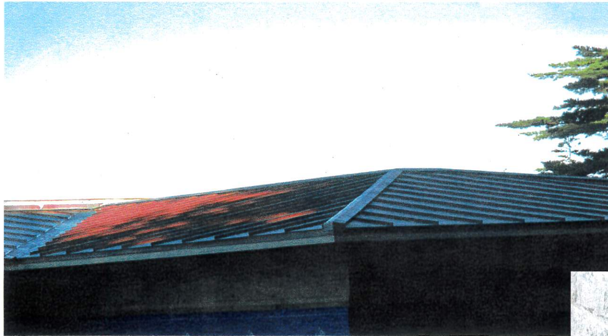
COPPER STANDING SEAM ROOF
