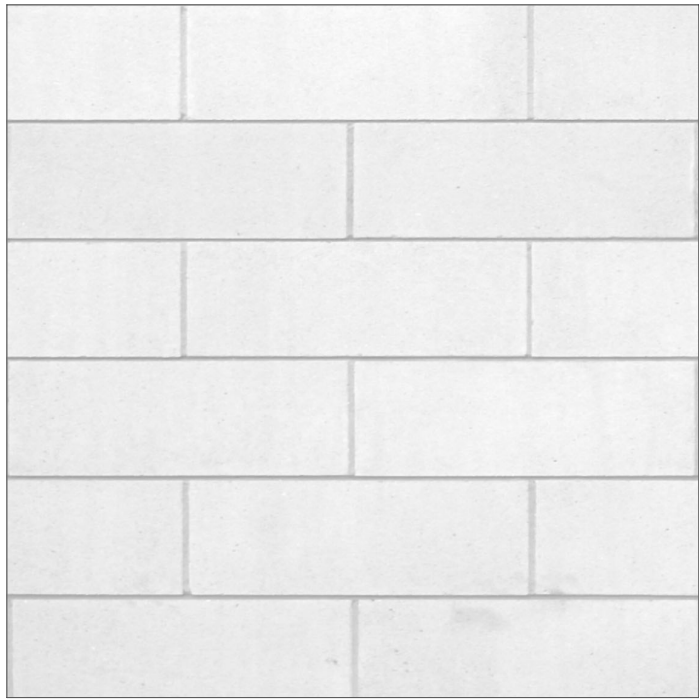
2 EXPOSED CONCRETE MASONRY UNIT (CMU) BLOCK - 4"X16"X8"; SMOOTH 'SACKED' WHITE-WASH PLASTER FINISH
