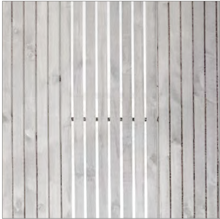
10 VERTICAL TIMBER WOOD SCREEN - 2X WD. BOARDS SPACED 4" O.C.; WHITE-WASH FINISH TO MATCH WOOD SIDING
