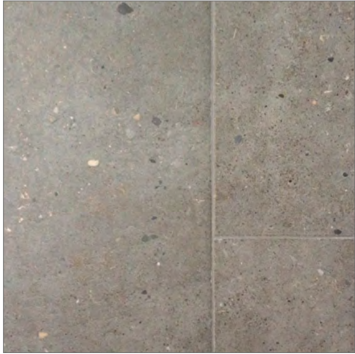
4 BRUSHED SEVILLE LIMESTONE; EXTERIOR PAVING AND DECKING
