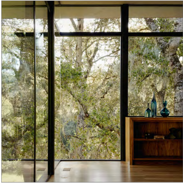
7 ALUMINUM EXTERIOR DOORS & WINDOW FRAMES - THERMALLY BROKEN; DARK-BRONZE ANODIZED COLOR
