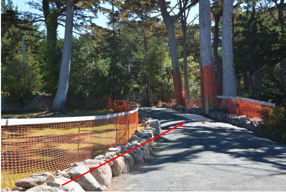
Note plywood to protect roots
