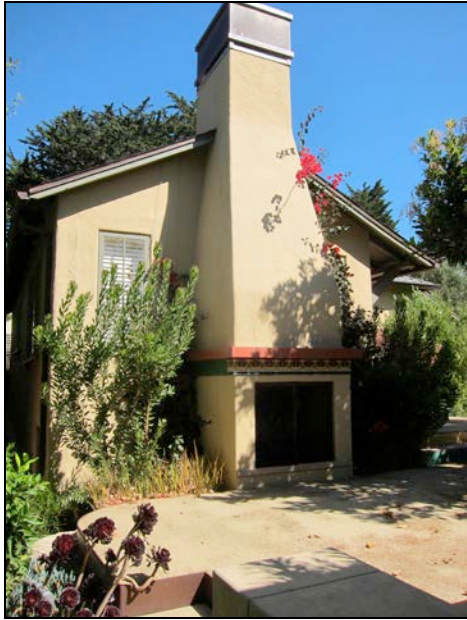
Figures 3 and 4. Left image shows the front elevation of the guesthouse, with large front chimney with newer stucco cladding and chimney cap. Right image shows the front elevation of the guesthouse.
