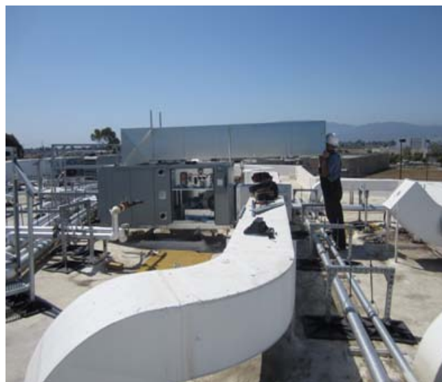
Photo 3-1. HVAC System Retrofits Being Installed at the County Jail
