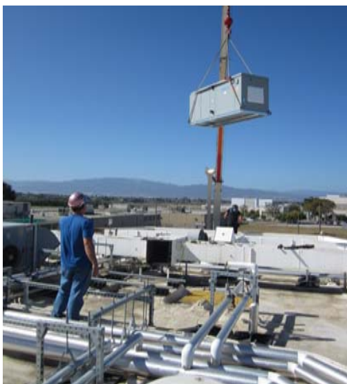
Photo 3-1. HVAC System Retrofits Being Installed at the County Jail
