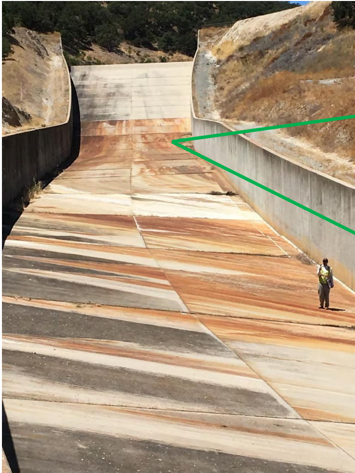
Upstream Portion Spillway Chute
