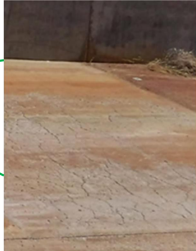
Concrete Degradation due to Groundwater Seepage
