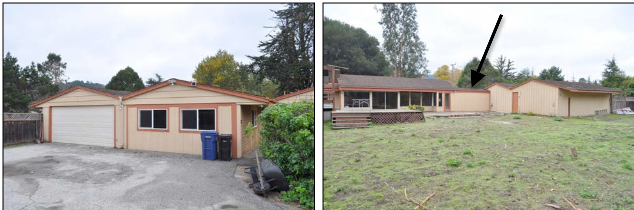
Figures 3 and 4. Left image shows the original four-car garage, with half of the structure converted to living space with windows added in 1993. Right image details the rear elevation, showing substantial fenestration modifications and connection of the garage to the house via a breezeway (arrow).
