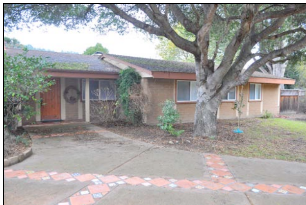
Figures 1 and 2. Left image shows the front elevation taken from the driveway. The large gable-roofed mass with board-and-batten wall construction was constructed in front of and connected to the house in 1993. Right image shows the remaining post-adobe portion of the front elevation, with replaced front door and replaced windows.
