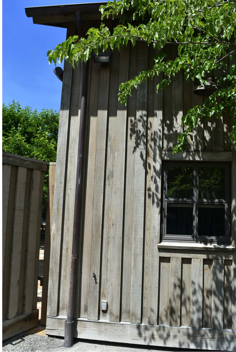
'WEATHERED WOOD' BOARD AND BATTEN SIDING & BRONZE ANODOZIED CLAD WOOD WINDOWS/DOORS
