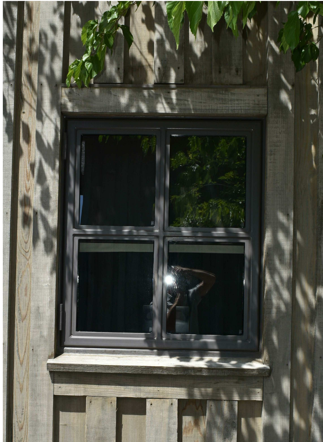
'WEATHERED WOOD' BOARD AND BATTEN SIDING & BRONZE ANODOZIED CLAD WOOD WINDOWS/DOORS
