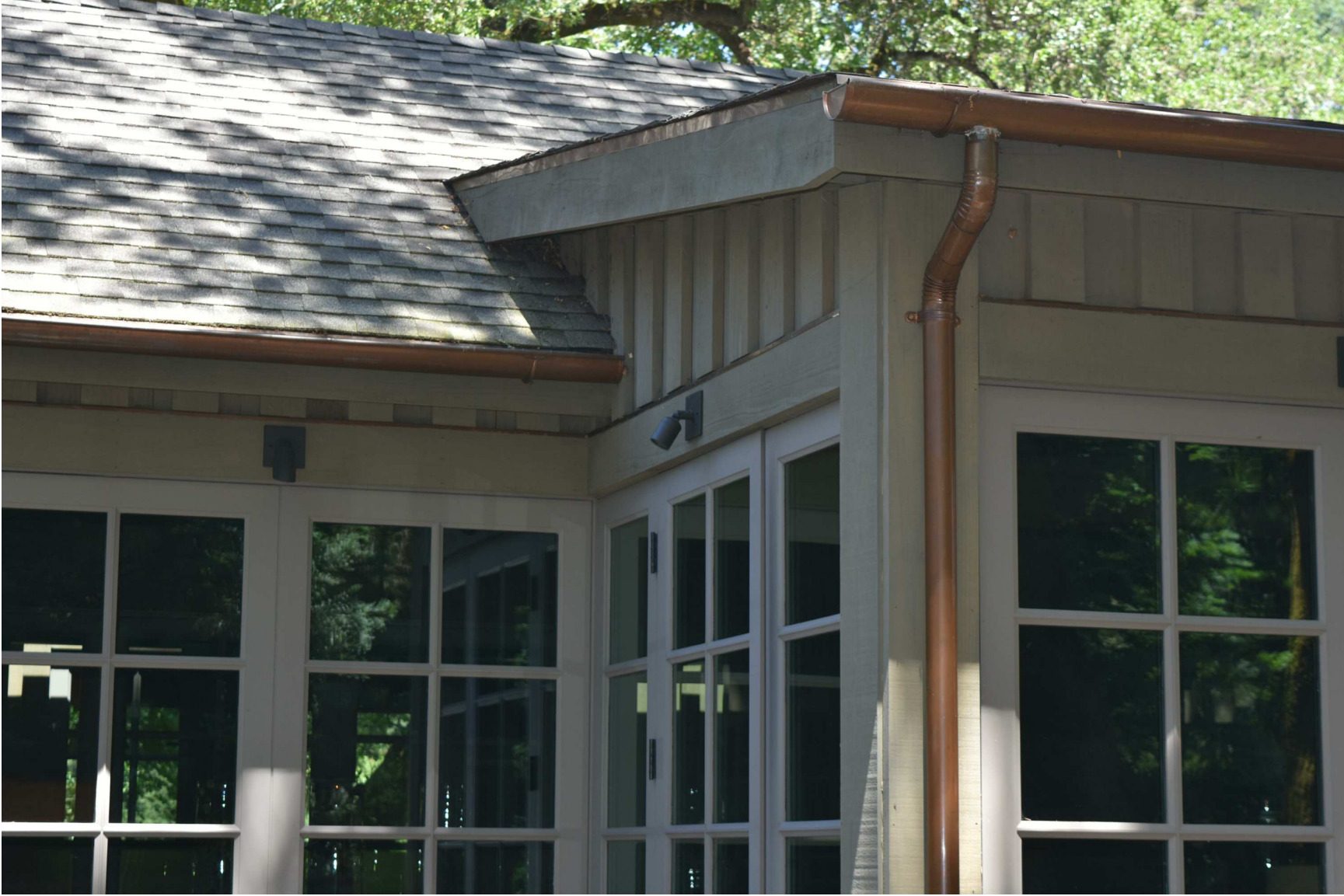
COPPER GUTTERS & DOWNSPOUTS AND HEAVY PROFILE COMPOSITION SHINGLE ROOFING
