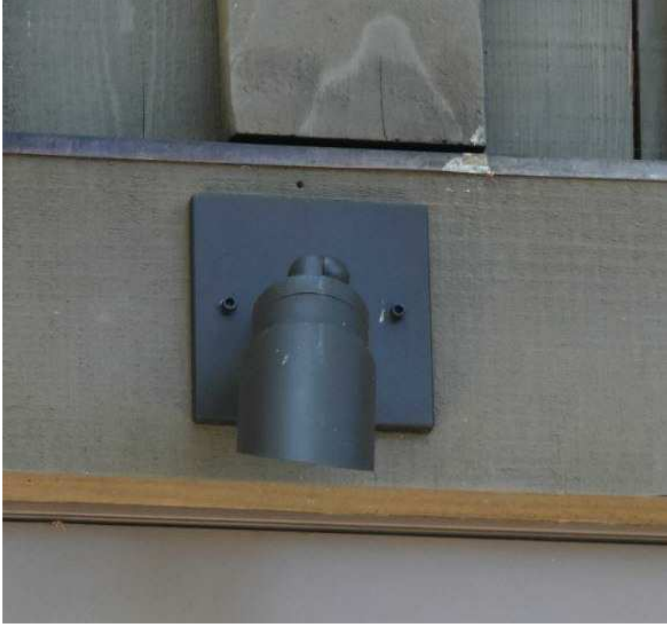
EXTERIOR DOWNLIGHT & COPPER HEAD FLASHING AT OPENINGS
