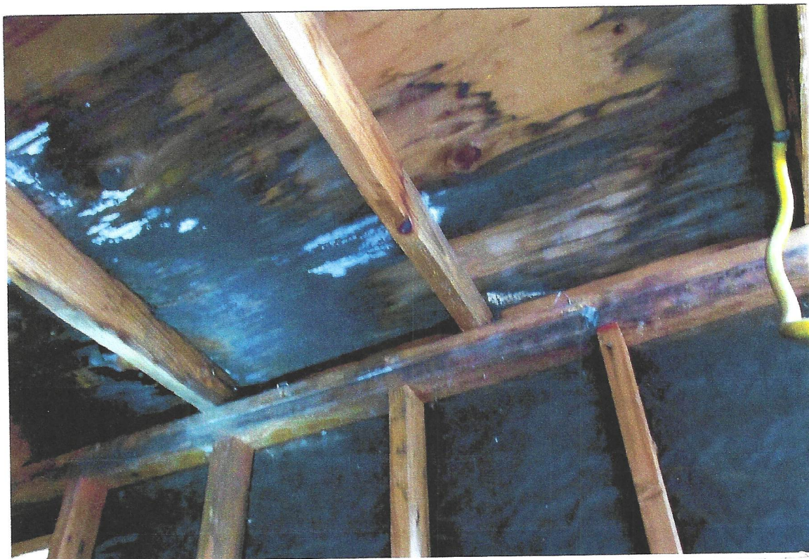
Photo #3. Looking at interior ceiling mold, found throughout bldg. Kent Seavey, June, 2022.
