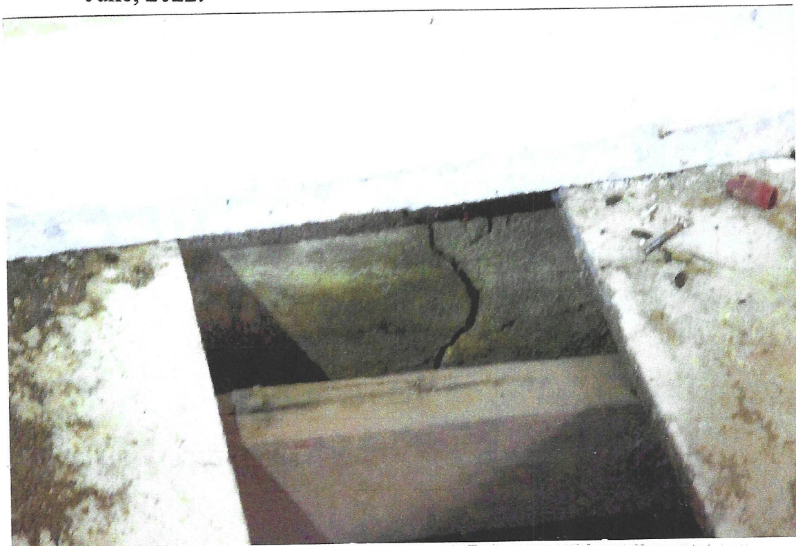
Photo #4. Looking at typical cement foundation failure in living room, Kent Seavey, June, 2022.
