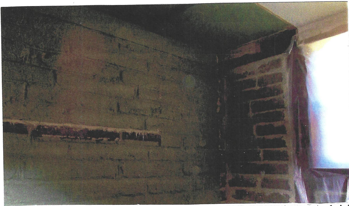
Photo #2. Looking NW at interior wall cladding, note single wythe adobe brick and use of cement mortar, Kent Seavey, June, 2022.
