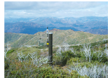
Flood warning gage
