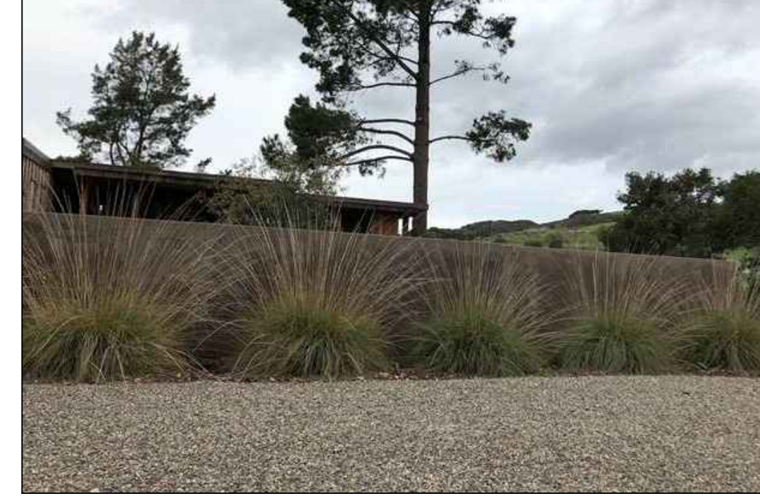
Concrete Retaining Wall
