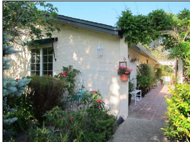
Figure 15. Bldg. 25 constructed of adobe.
