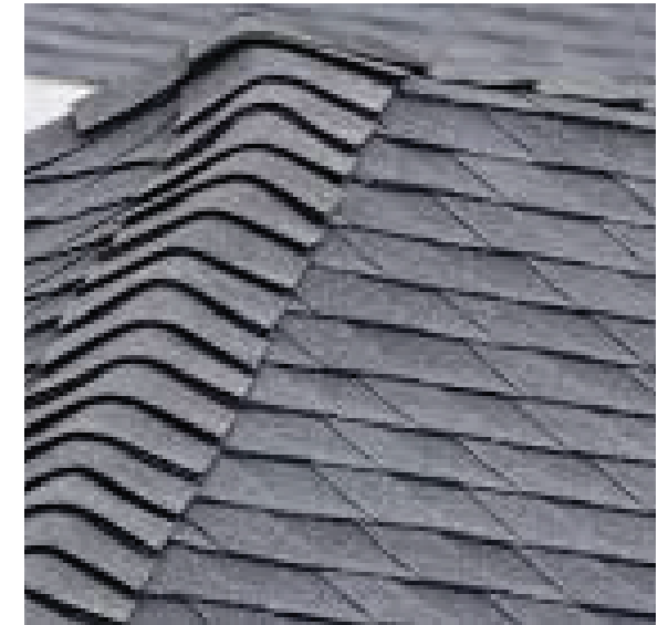
Roofing: Asphalt shingles to match existing
