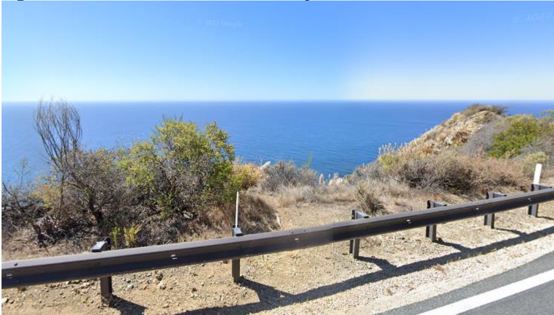
Figure 1-4 Stained Midwest Guardrail System
