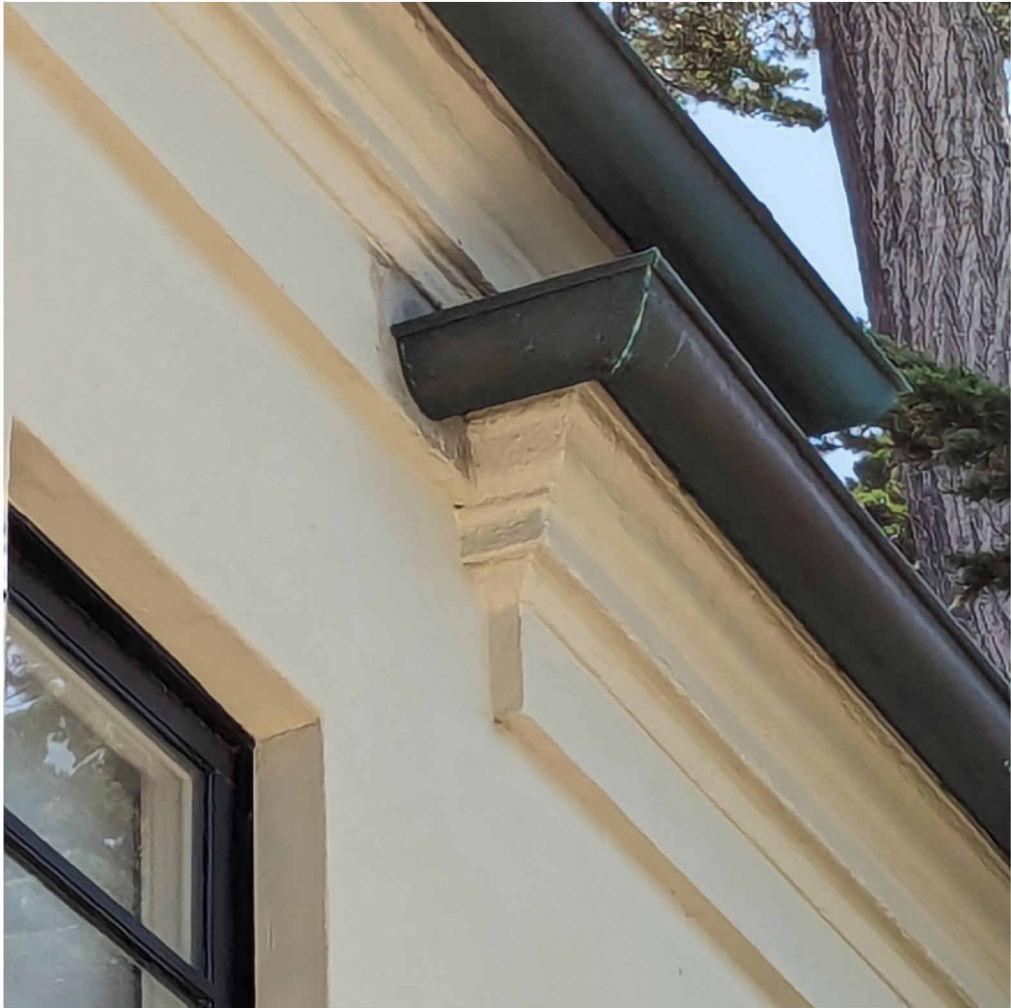
(E) COPPER METAL GUTTER & RWL
