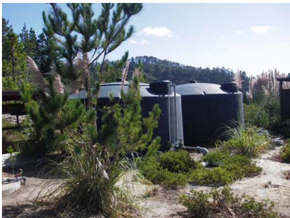
Photograph 3. Project site, looking south at existing water tanks to be demolished.
