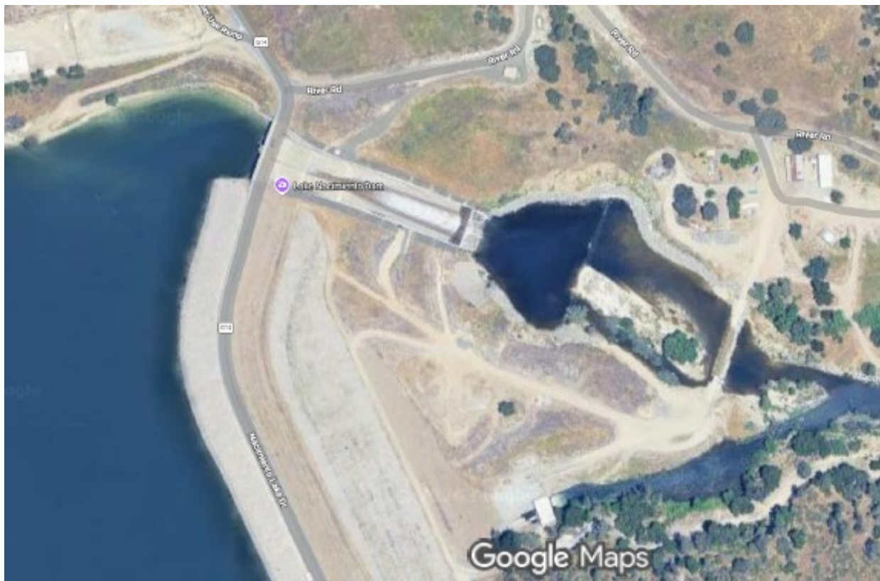
Figure 3: Nacimient Dam Spillway Plunge Pool
