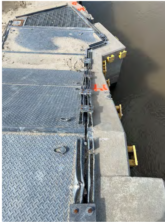
Bent Fish Ladder Top Panels (Three panels damaged)
