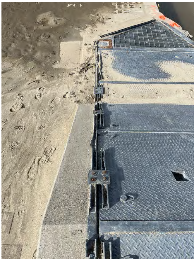
Bent Fish Ladder Top Panels (Three panels damaged)
