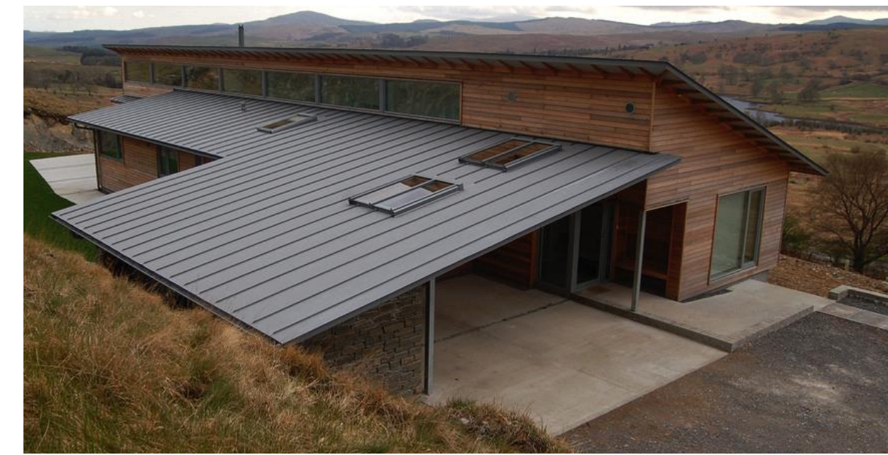
M2 GREY STANDING SEAM METAL ROOF
