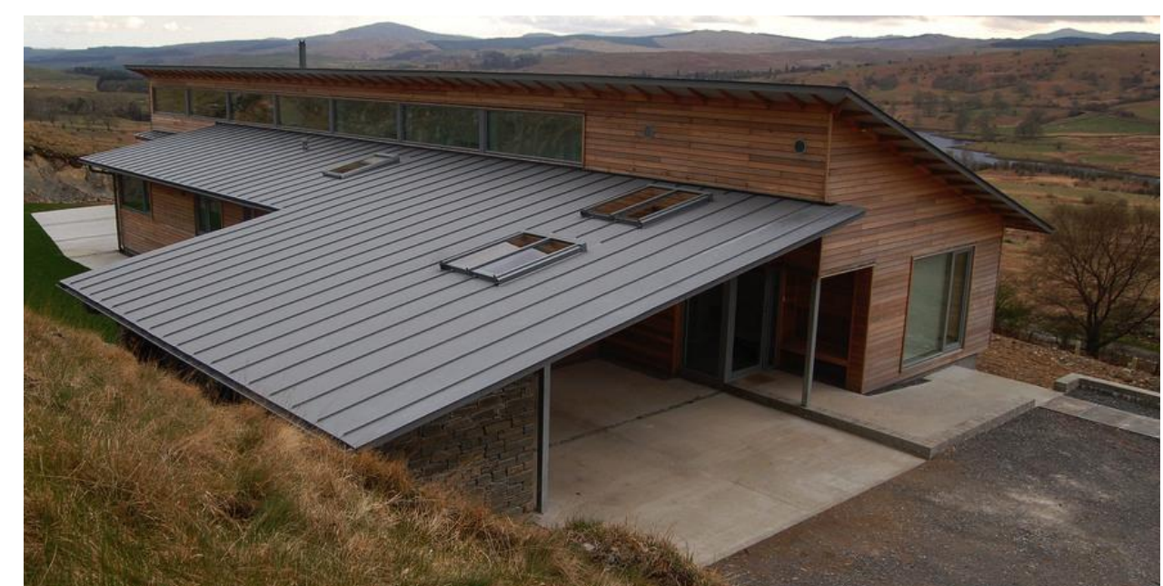
M2 GREY STANDING SEAM METAL ROOF
