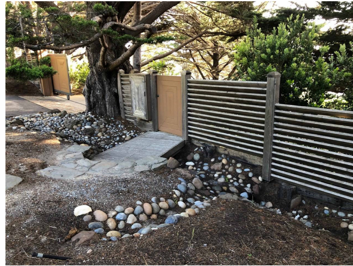
ACCESS DOOR AT MAIN ENTRY GATE
