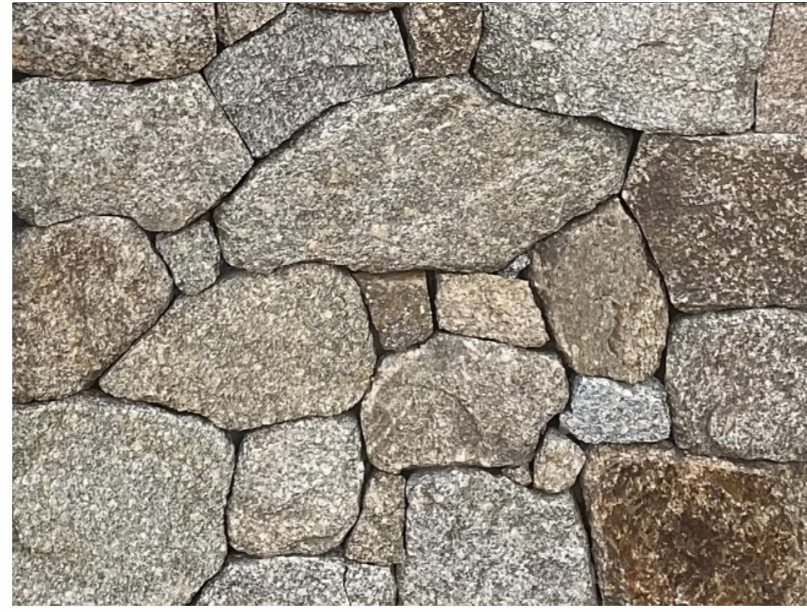
LOCALLY SOURCED, UNCOURSED RANDOM ASHLAR STONE WALLS
