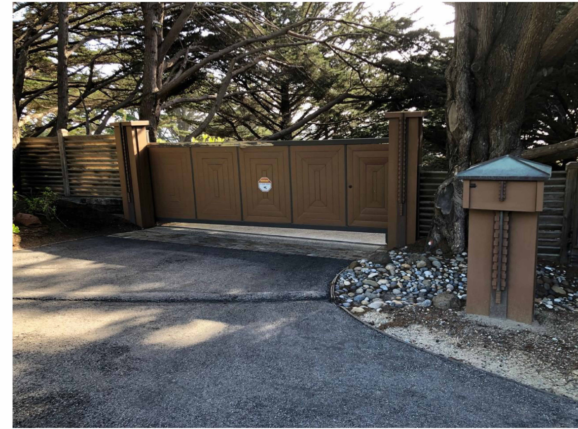
MAIN ENTRY GATE
