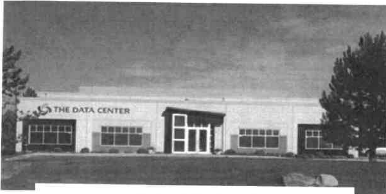
Front View of the Data Center
