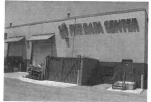
Rear Entrance to The Data Center
